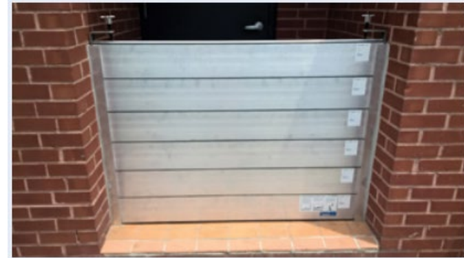
The newly-installed flood gates over entryways. Image: Services for the Underserved.
