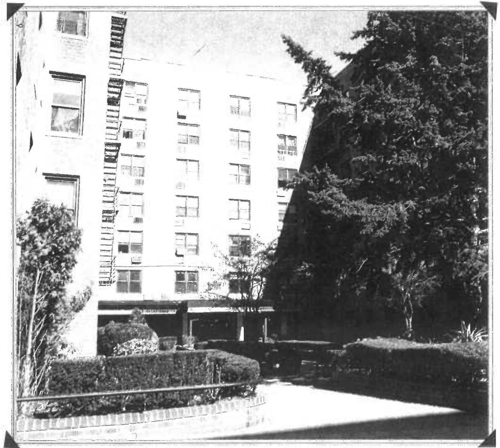
Atlantic Towers in the Sheepshead Bay section of Brooklyn is one of New York City's most well-appointed affordable cooperatives. A $11.3 million loan, insured by SOFHYMA, has brought this housing back to financial stability.
